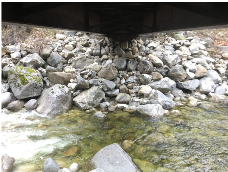
Left Bank Abutment when facing downstream
