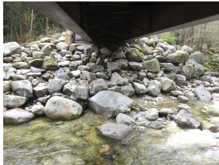
Right Bank Abutment when facing downstream
